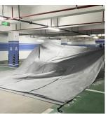
Pull off the fire blanket and completely cover the vehicle
